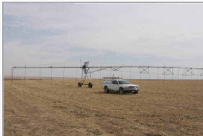
Figure 1 Installing a pivot control box.
